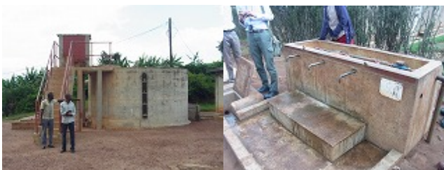
Photo 1 : Water storage tank (left), public-tap stand (right)
