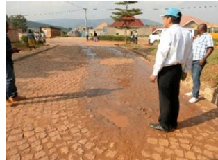
Photo4: Underground and Surface Leakage
