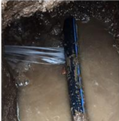
Photo4: Underground and Surface Leakage
