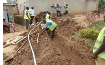
Photo7: Replacement of Distribution Pipe
