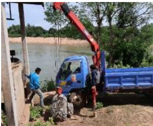
Installing motor after overhauling
