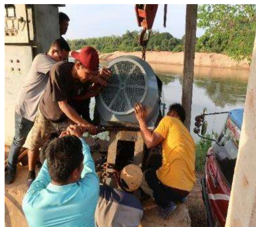
Installing motor after overhauling
