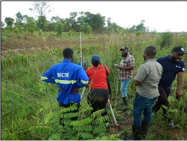
The picture shows candidate site investigation in Serenje district. Investigated items such as stream water volume, geographic condition, and vegetations are used for designing. (Serenje district in Central province)
