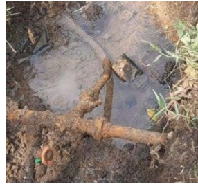
Photo 9 Example of leakage found through leak detection survey.
