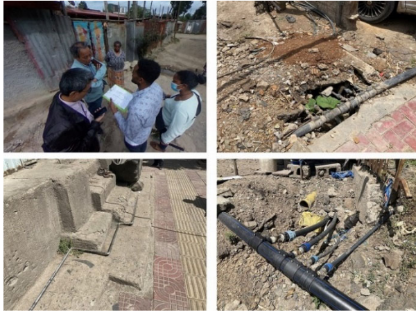
Photo 1 Situation of exposed piping and spaghetti pipes
