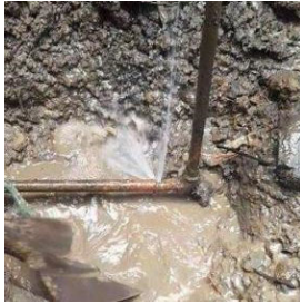
Photo 9 Example of leakage found through leak detection survey.
