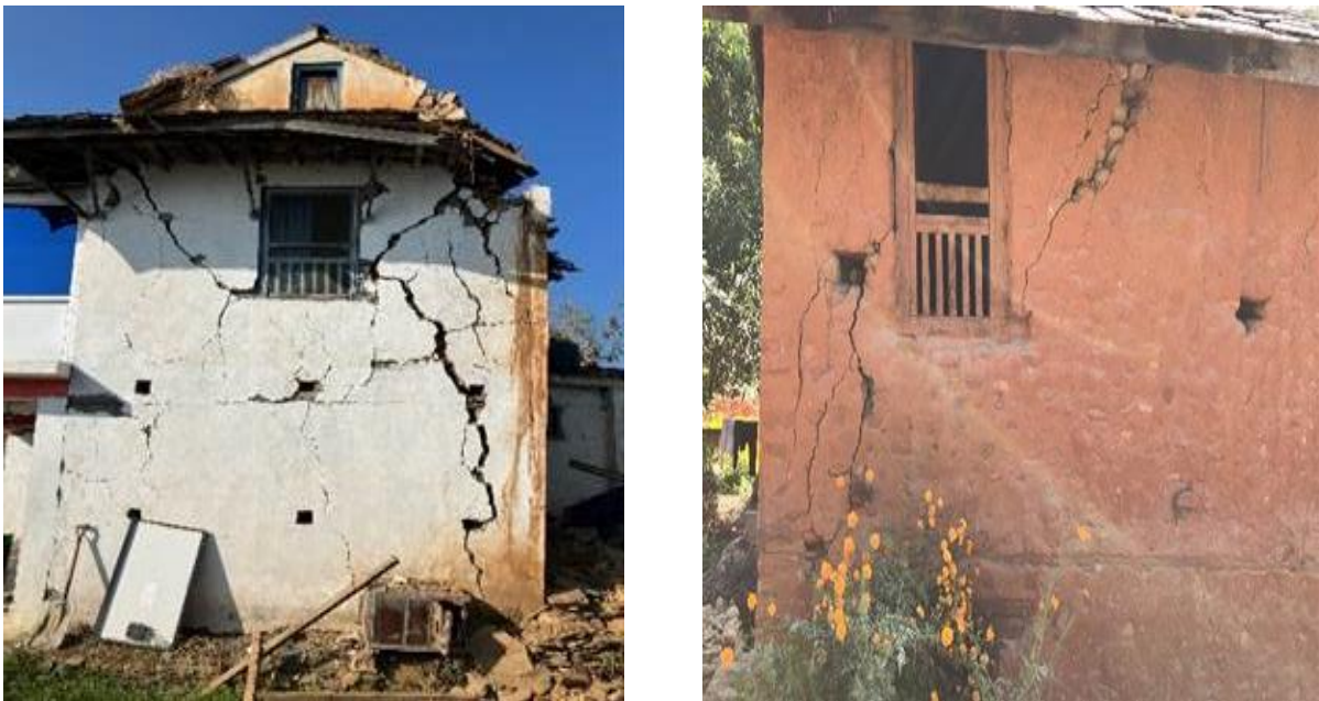
Figure 4: Diagonal cracks
