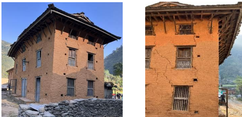
Figure 7: Vertical crack in opening
