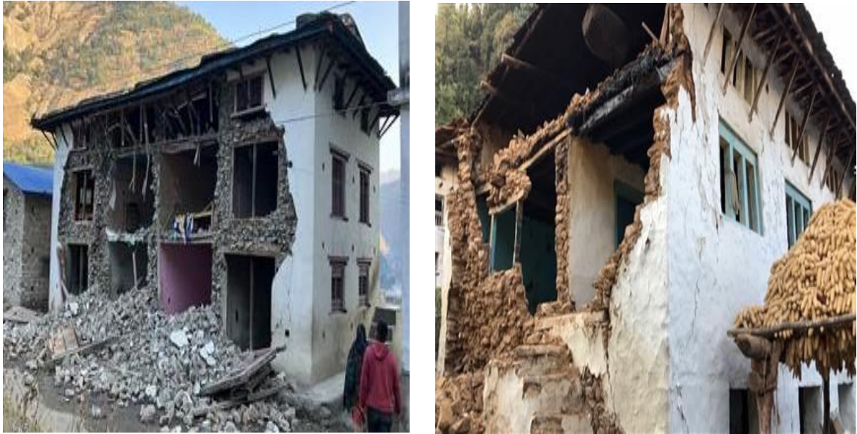
Figure 3: Out of plane failure
