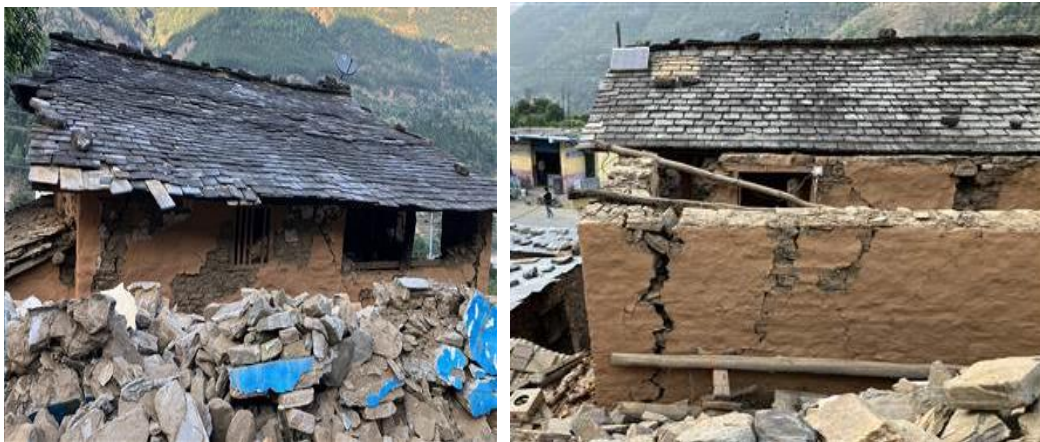
Figure 6: Building with heavy roof weight.
