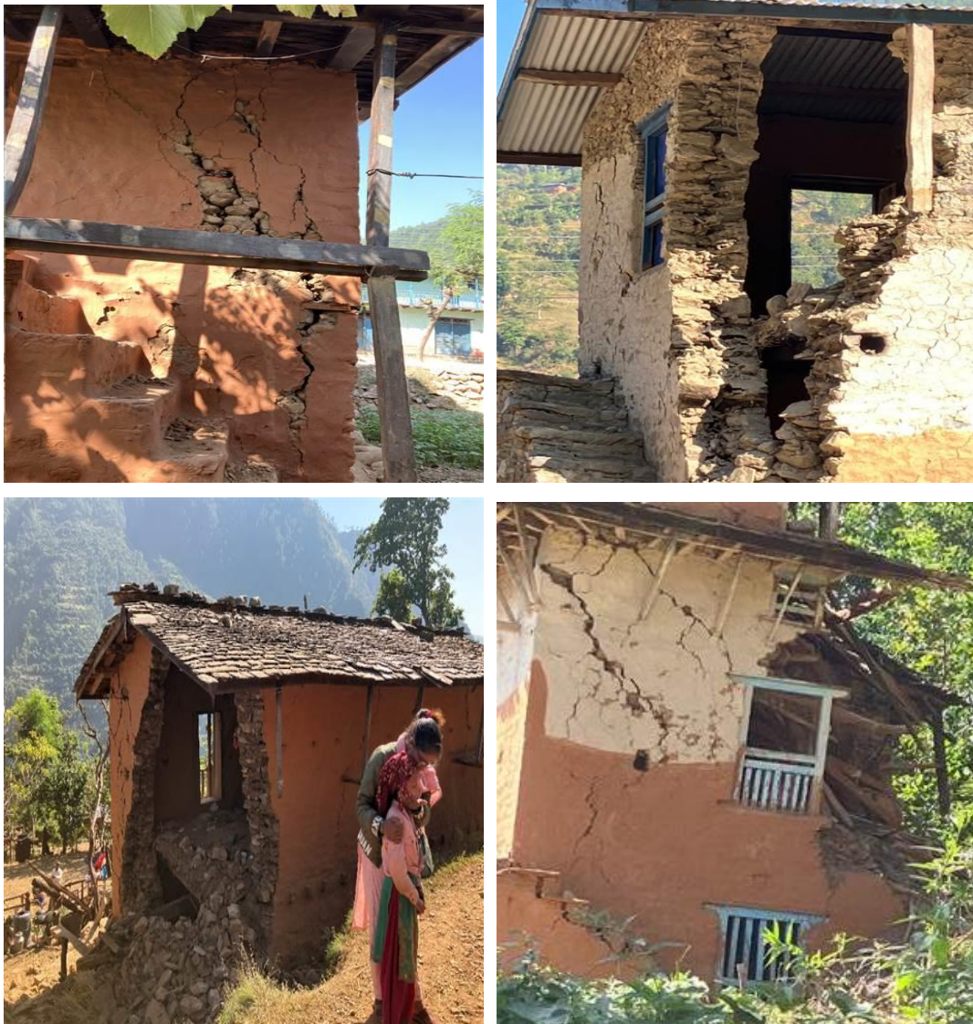
Figure 5: Corner failure
