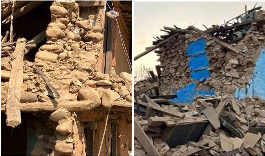
Figure 2: No through stone block in wall thickness
