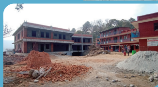
Surveying target sites
