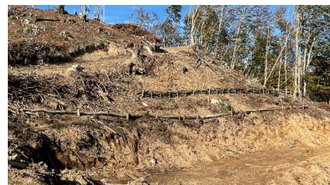
Log erosion barriers (LEBs)
