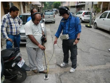
Technical Assistance for Leak Detection
