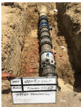
Valve and Flowmeter installation
