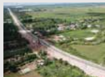
National Road No.5 Improvement Project (Photo: TEKKEN CORPORATION)
