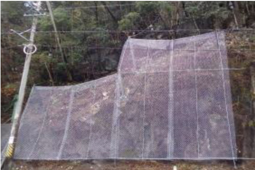
Pocket type rockfall prevention net work
