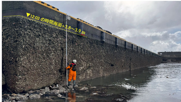
Port Warf rose 4m by ground upheaval
