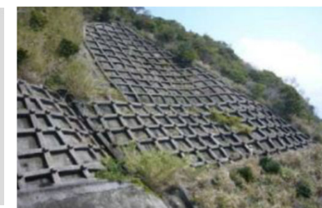
Frame work + Anchor work
