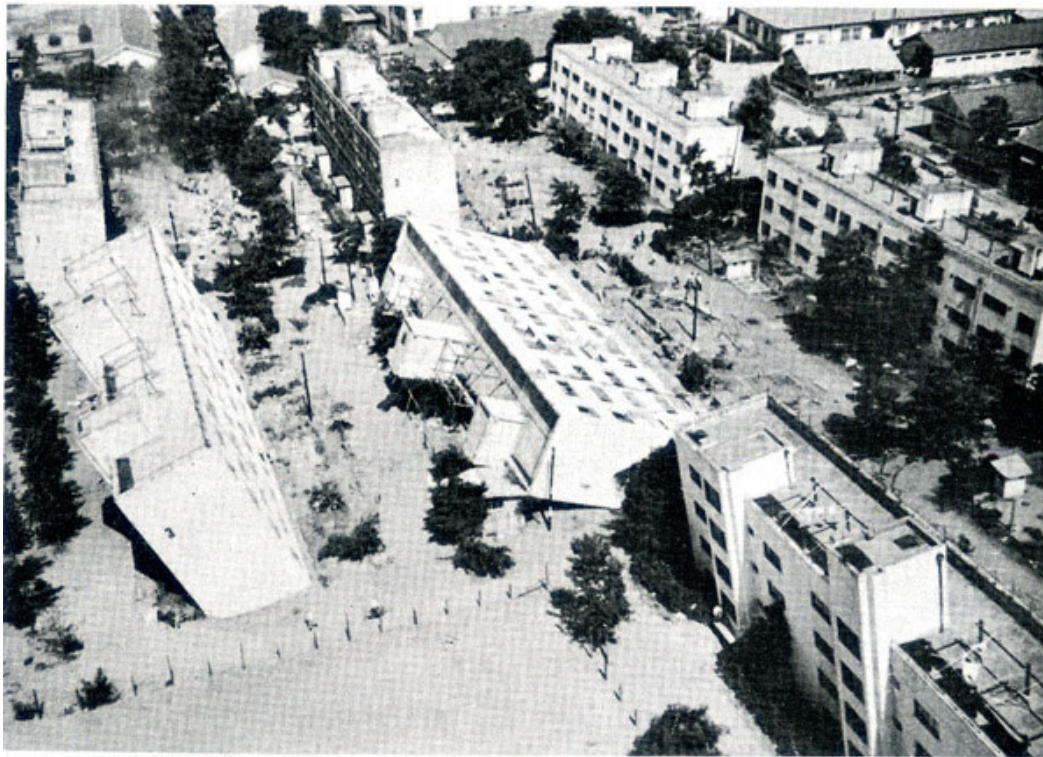
1964 Photo of RC apartments tilted by Ground Liquefaction
