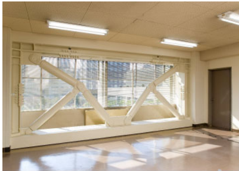
Seismic Brace with vibration damper inserted.
