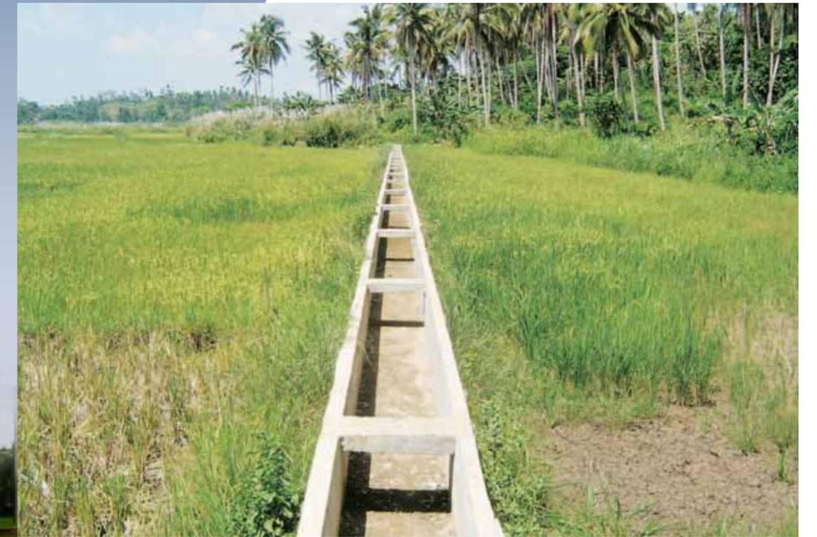
Rectangular canal with concrete hollow block sidewalls
