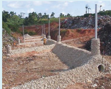
Construction phase of dumping site using FUKUOKA method
