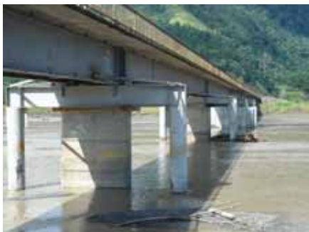
Strengthening Piers No1 to No4
