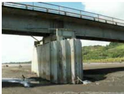
Condition of Pier No3
