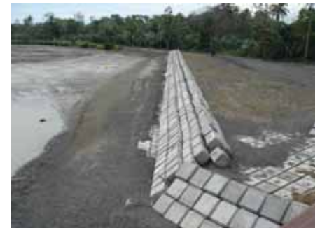
Lae side Bank Protection
