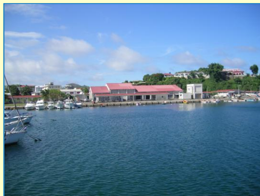
Cold storage facility in Vieux Fort Fishery Complex
