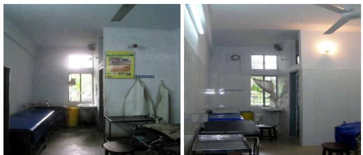
Before and after renovation of Polash UHC
