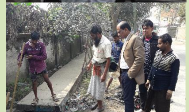
Observing Drainage Cleaning (CoCC)
