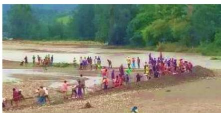
The river course in Buluto changed away from the intake side. Therefore, many farmers tried to remove sedimentation manually to divert water from the opposite side to the side of intake. The Project will continue to support the farmers and Water Users' Association (WUA) to coordinate with Ministry of Agriculture and Fisheries (MAF) national or local authorities to solve this challenge.
