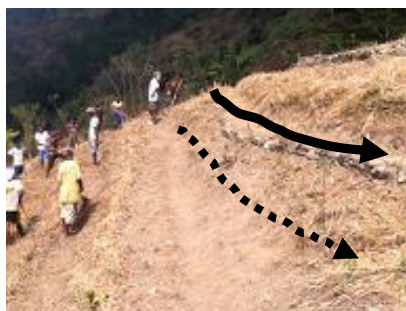
The contour line is not correctly delineated as the lines were taken without clearing the areas.
