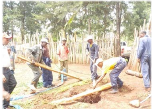
4. Cleaning the well and surrounding and make dewatering
