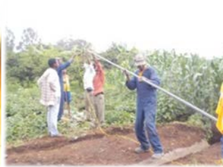
10. Putting pistons with rope in the raiser pipe
