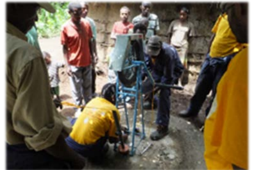
13. Inspection and adjusting of outlet pipe position
