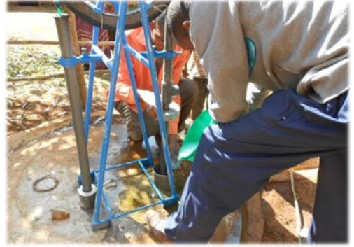
15. Disinfection of the well
