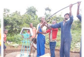
11. Inserting the raiser pipe in to the well
