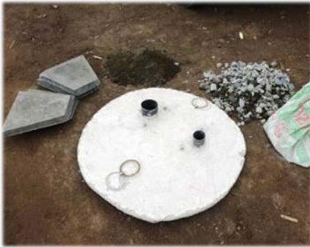
3. Preparation of materials; construction materials, pump accessories and working materials
