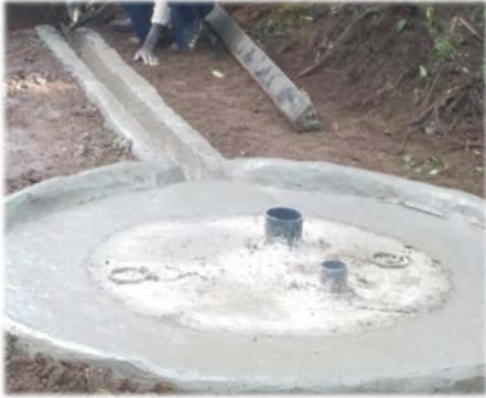
7. Finishing apron with concrete sealing
