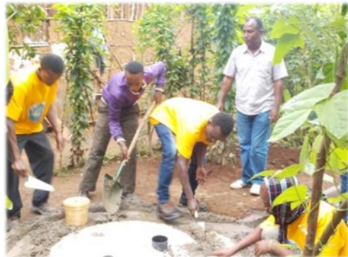
6. Placing a well cover on the reducer blocks
