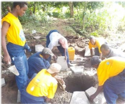
5. Construction of apron, putting reducer blocks and construction of drainage canal
