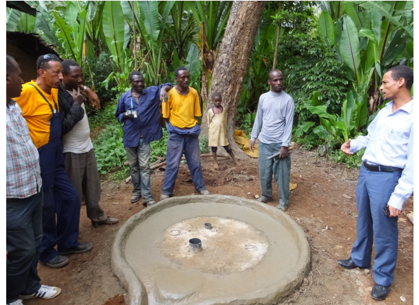
Installation of Rope Pump by trained Village Technicians (Yirgachafe woreda)
