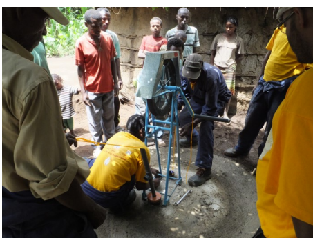
Installation of Rope Pump 7
