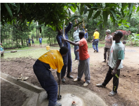
Installation of riser pipe 6
