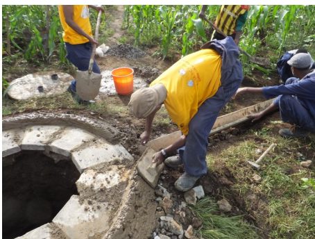
Construction of apron, drainage canal and soak away pit 3
