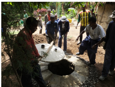
Placing of well cover 4
