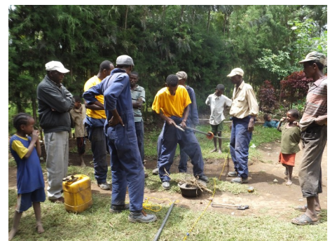
Preparation of riser pipe, rope and pistons 5
