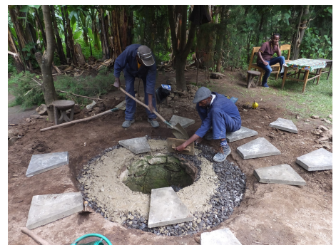
Setting of reducer blocks 2
