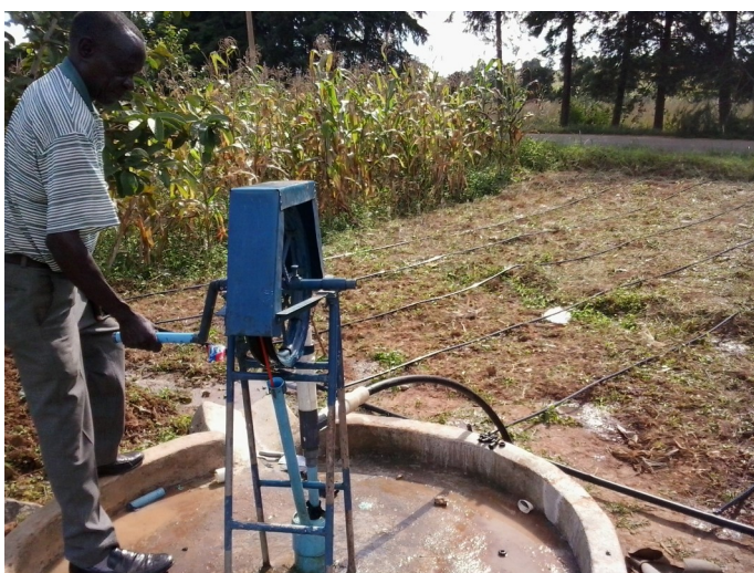
Practice of small scale irrigation (water distributed through closed pipe system with gravity)
