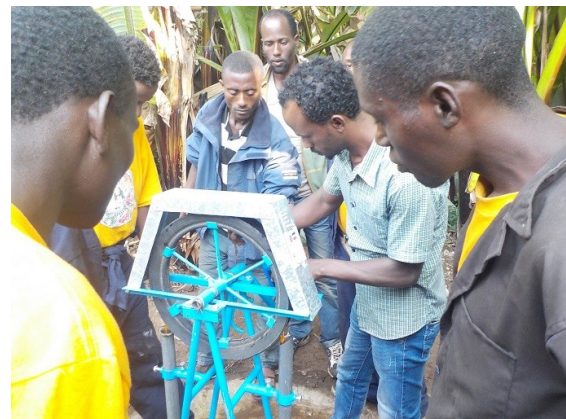
Quality check after installation by Mr. Alene, Technical Assistant of JICA WAS-RoPSS (center) (Photo by WAS-RoPSS)
