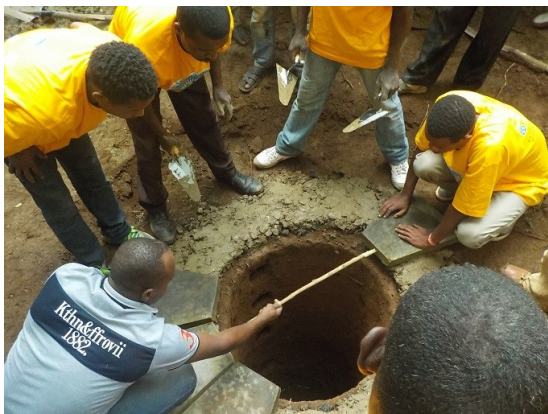
Installation of reducer blocks, taught by TVETC instructor, Mr. Tarekegn (front left) (Photo by WAS-RoPSS)
