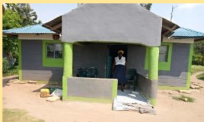
Ms. Monica's newly built house
