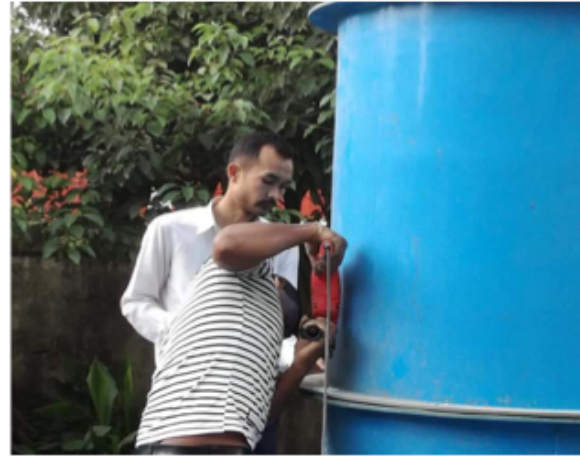
Figure 3.7. Radial drilling to connect main body of nitrification unit
