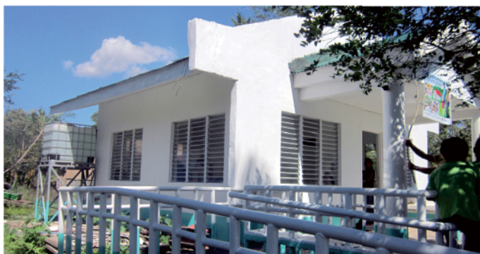
Figure 1: The LGUs of Luna undertook the renovation of BHS Marag
