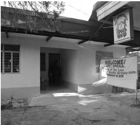
Newly Renovated Delivery area of Luna RHU
