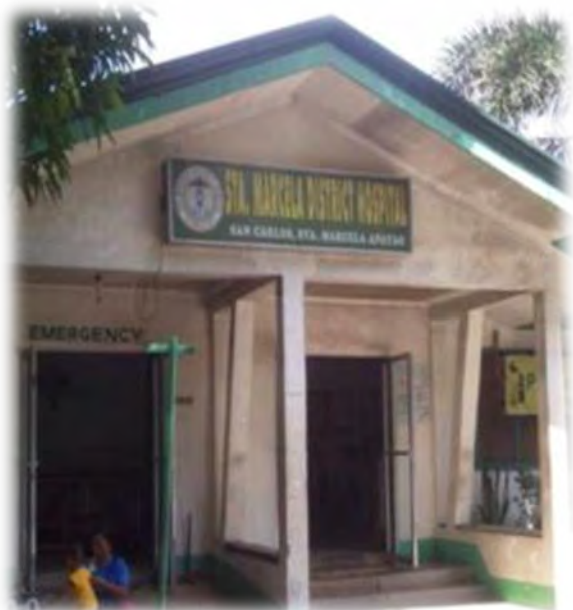
Sta. Marcela District Hospital
