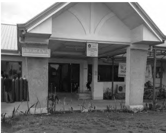
Entrance of the Emergency Room (FNLGHTC)
