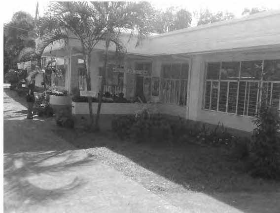
Side View of the District Hospital (AJDH)
