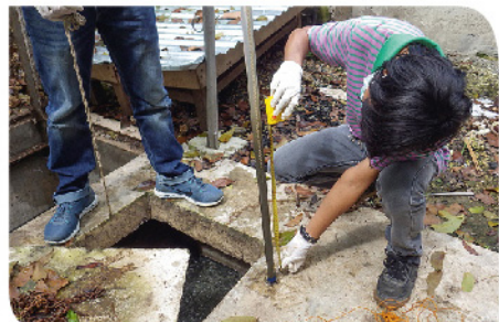
Measuring sludge depth
