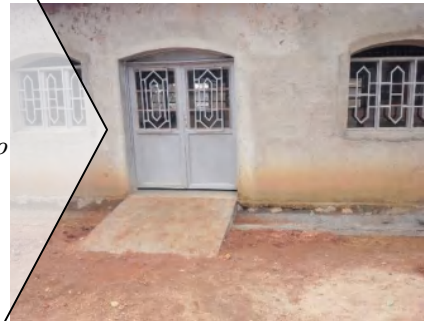
Before and after barrier-free construction in VTC Nyanza Mbere na nyuma yo kuvanaho nzitizi ku bafite ubumuga
