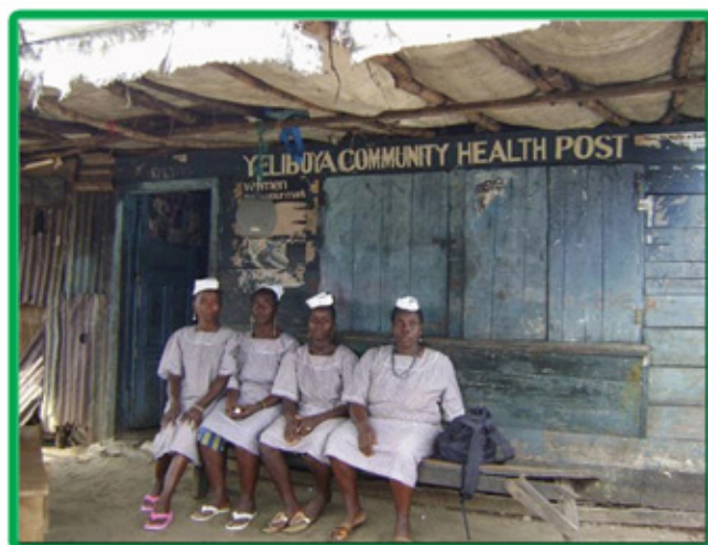
Present Yeliboya PHU constructed by community
