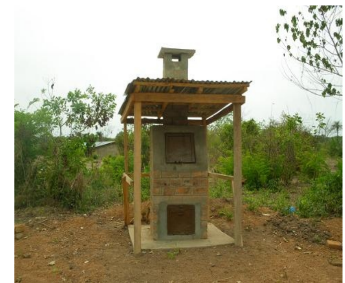
A New Incinerator at Konta PHU
