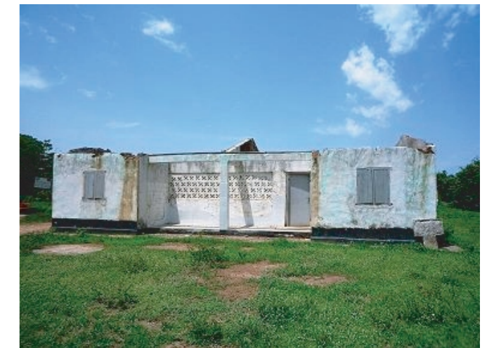
Konta PHU before rehabilitation
