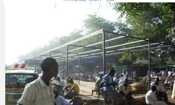
Constructing the skeleton for direct sale place.
