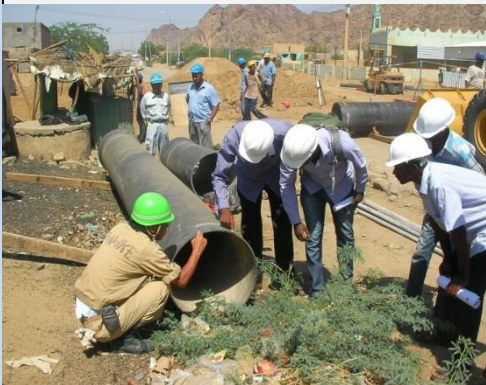
SWC engineers ask about the pipe materials.
