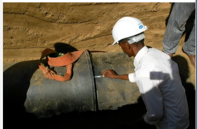
The SWC engineer checks the quality of connection using a gauge.
