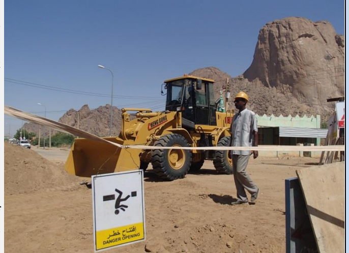
Safety assessment methods in the construction site
