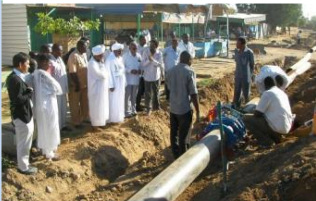
Commencement ceremony for the water pipe replacement work.
