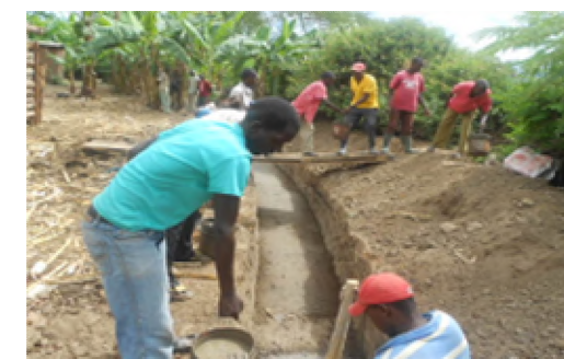
Dissemination II : Canal Construction at Kyamakata scheme in Meru district
