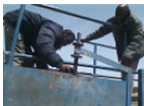
IO members are maintaining an intake gate according to the maintenance plan at Ijinga scheme, Mwanza zone
