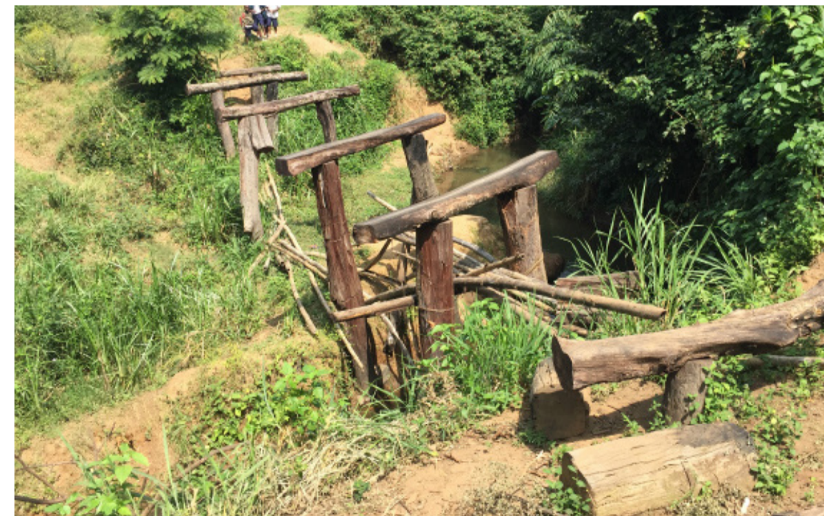
Construction of Community Bridge continues for finishing in 2019.
