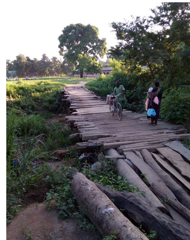
Villagers in Mshikamano started to construct Community Bridge in 2016 and now utilize the bridge for economic activity and receipt of the education in nearby village.
