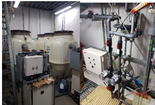
Photos showing Jokasou with gas emission measurement facilities
