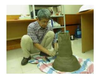
Local materials such as clay can be used to make a combustion chamber
