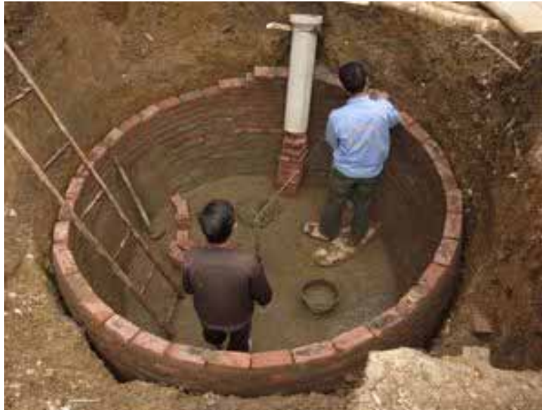
Construction of Brick-type biogas facilities in Tia Ghenh C
