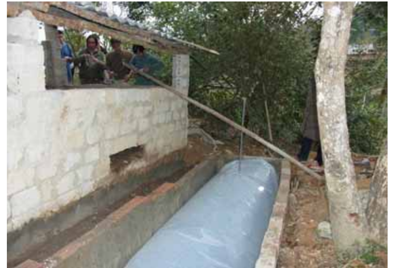
Polyethylene (PE) - type biogas facilities in Sai Luong Village
