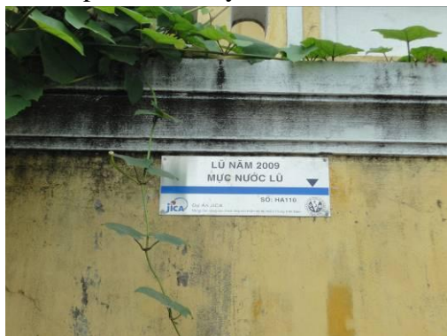
Installed Flood Mark Pates
