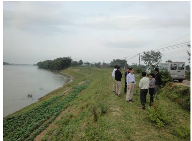
River bank protection pilot site (Quang Nam)
