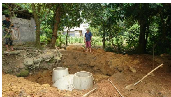
Image 20. Supervision of Biogas plant installation by Mr. Nguyễn Lương Phu household (Ngoc Lai village)
