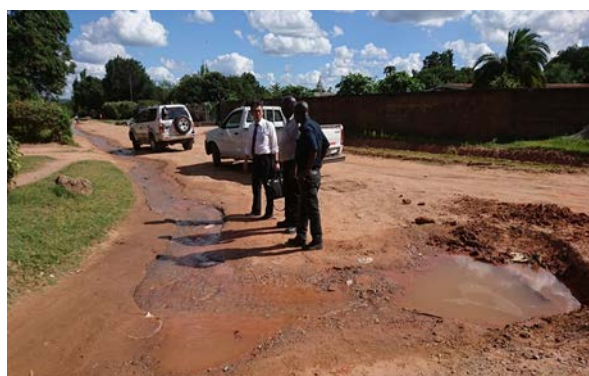
Picture-1 Surface Leakage in KWSC
