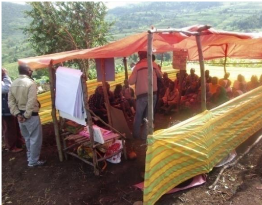
Figure24. Temporary roofing structure
