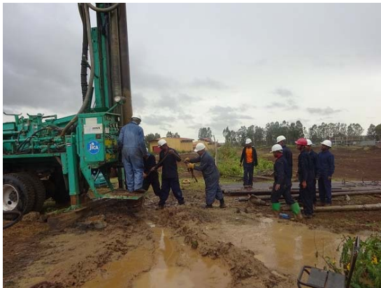
Photo 5: Drilling training at NRRTC
