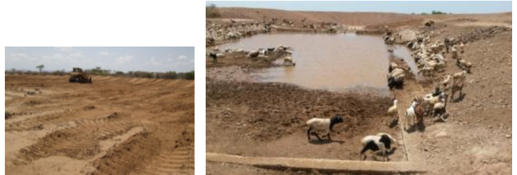
↑ Photo) Left: Bulldozer in Nachuro pan, excavating soil. Right: Nasikiria pan has standing water due to rain during construction.
