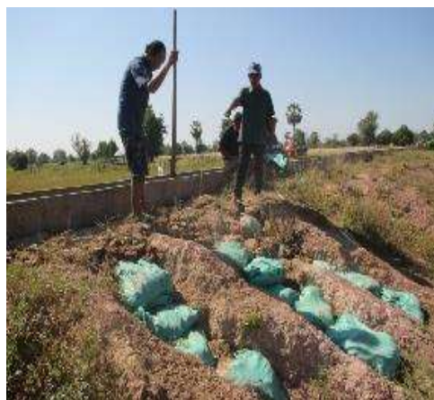
Put the sandbags in erosion part
