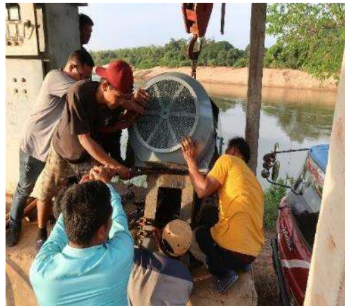
Installing motor after overhauling
