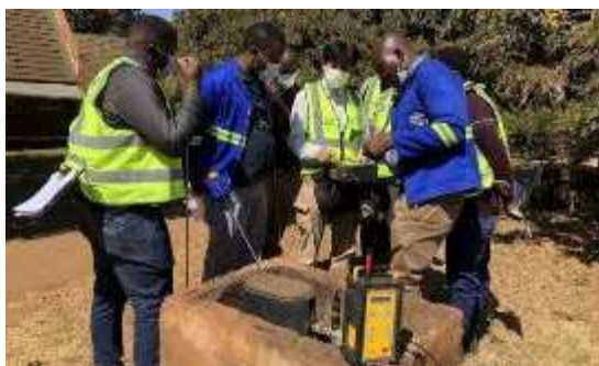
Photo 3: Training on Leak Detection
