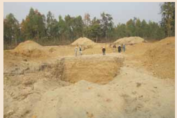
Dholan bridge, Mahottari
