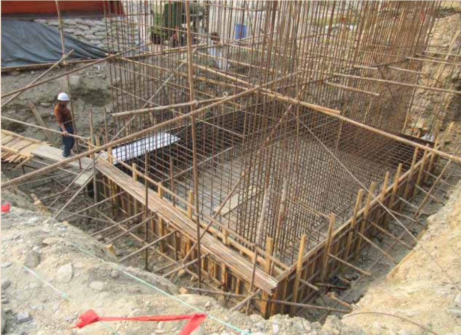
Bridge being constructed in Rosi River, Kavrepalanchowk
