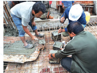
Collecting concrete cube sample
