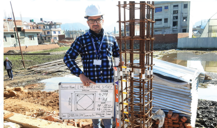
Supervision consultant must submit the photographic evidence as shown during the submission of supervision report
